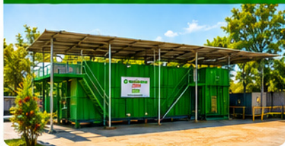
200 KLD DSTP INSTALLED AT YAMUNA VATIKA
