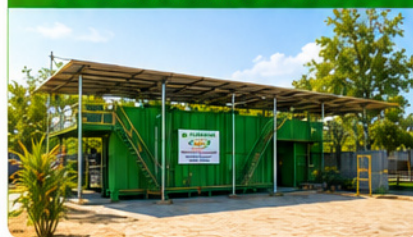
200 KLD DSTP INSTALLED AT YAMUNA VATIKA
