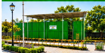
200 KLD DSTP INSTALLED AT SHUBROTO PARK
