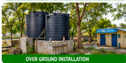
OVER GROUND INSTALLATION
