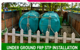
UNDER GROUND FRP STP INSTALLATION
